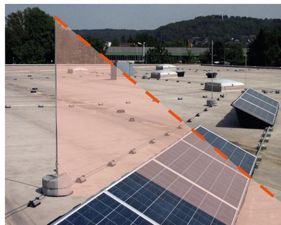
Figure 12 Determination of the protected volume using the protective angle method
